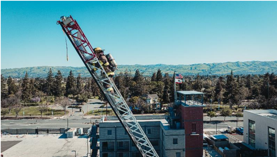
Fire Training Facility (Academy Ladder Training)
