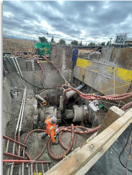
Martial Cottle Park Excavation
