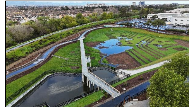
River Oaks Regional Stormwater Capture Project
