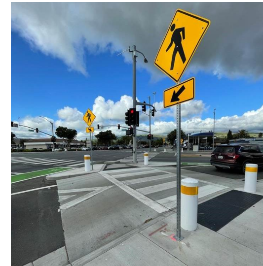
McKee Road Pedestrian Improvements
