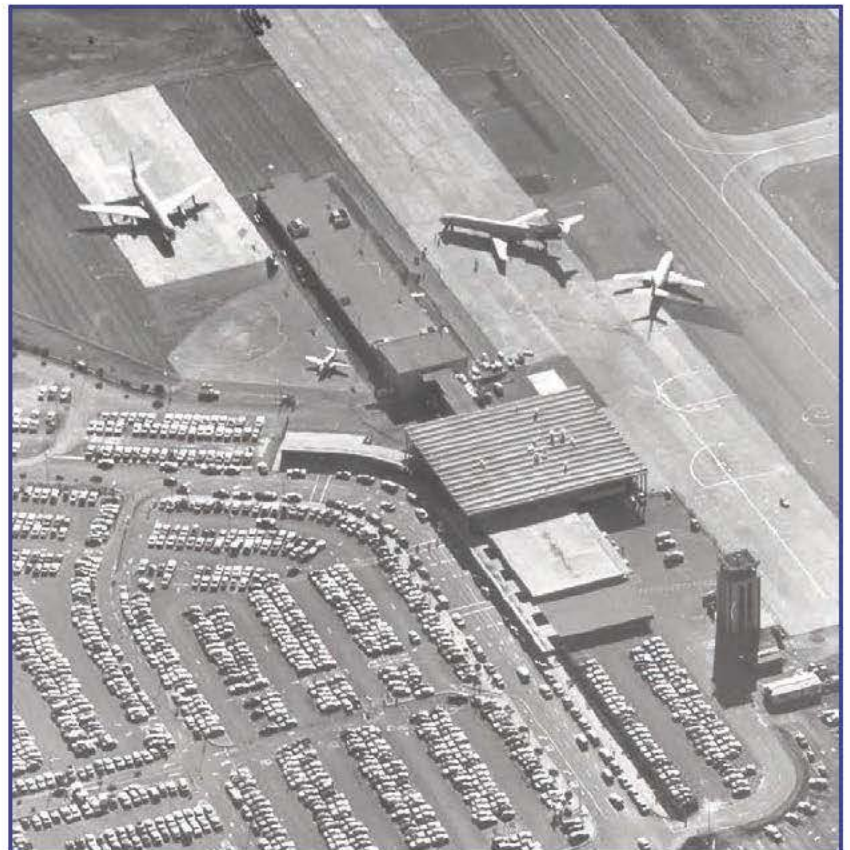
In August 1969, the airport opened a new six-gate extension on the south end of the terminal. Four months later, passengers board a PSA 727-200 flight as an Air California 737 headed for Southern California taxis away. A United DC-8 is parked at Gate 5. (SJC)
