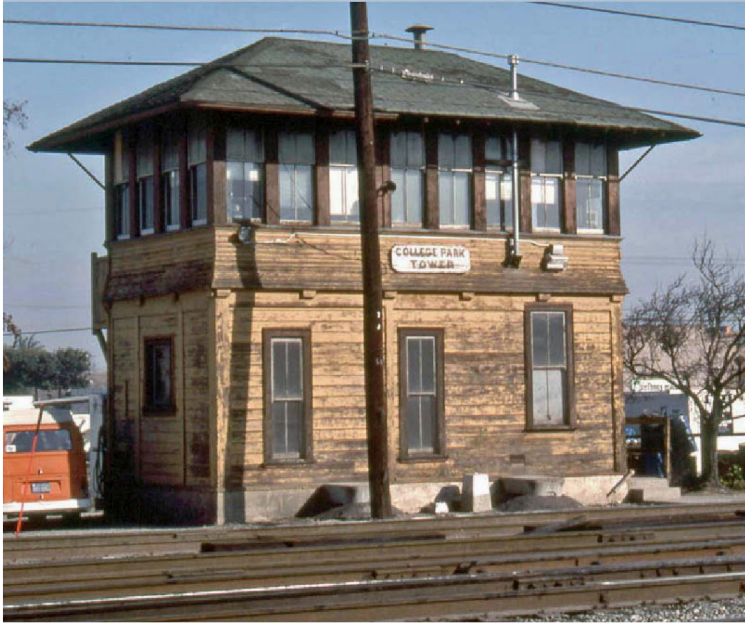
Figure 3: Southern Pacific Switching Tower (1980s photo courtesy of Willis Marshall)
