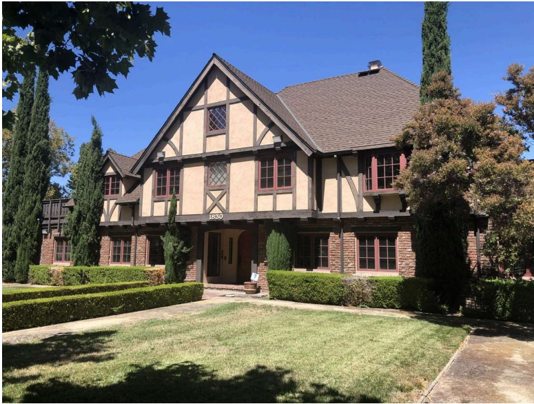
1060 Emory Street - Across the street from the project site.
