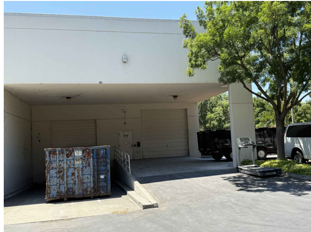
6 EXISTING BUILDING - NORTH N.T.S. FOR REFERENCE ONLY
