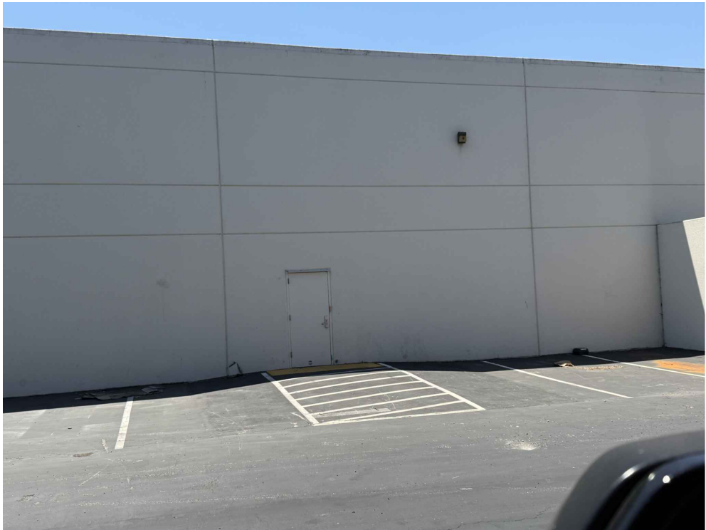
10 EXISTING BUILDING - NORTH N.T.S. FOR REFERENCE ONLY
