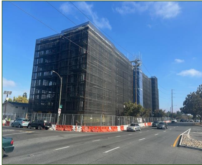
Image 25: The Charles project (99 affordable units) at 551 Keyes St (under construction)
