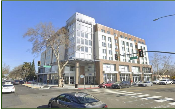
Image 7: Sparta student housing (construction complete in 2022)
