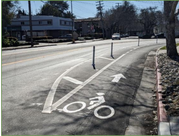
Image 10: Lane reduction and new bike lanes on Taylor St. implemented via pavement maintenance.
