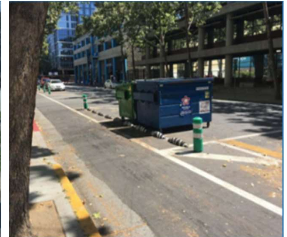
Curbing for dumpster set-out on San Fernando Street
