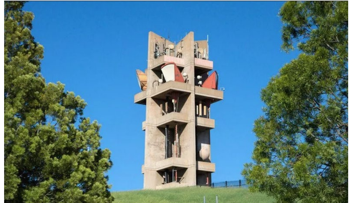
AT&T Tower, constructed 1972
