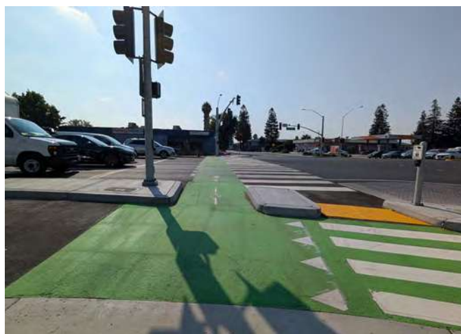
Recent crossing improvement of Trimble Road (looking south at De La Cruz Boulevard)
