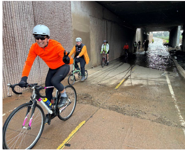
Figure 1: Flooded section of the GRT under Highway 237. (Image Source: Tim Oey)
