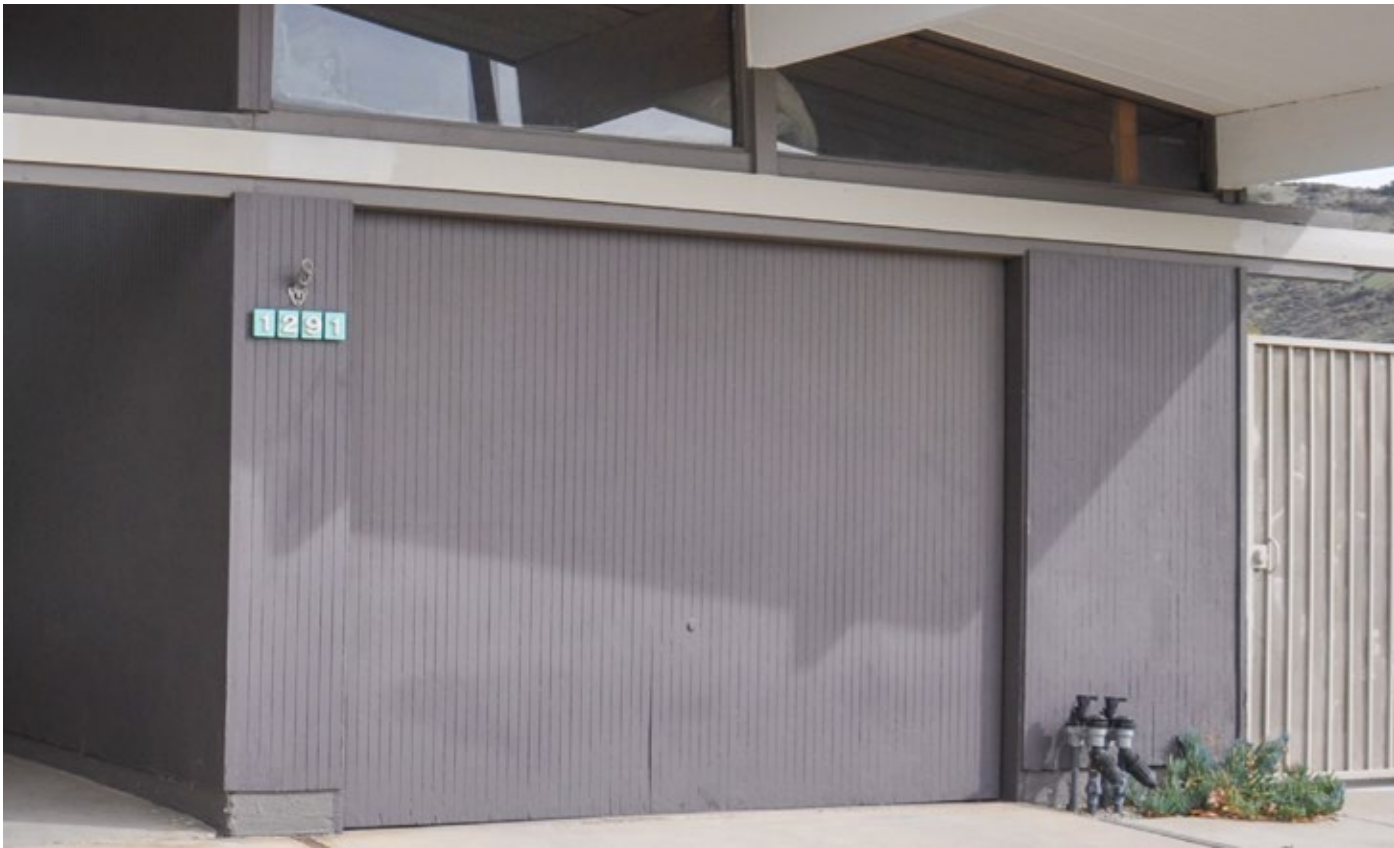
Figure 15: Original vertical groove plywood cladding.
