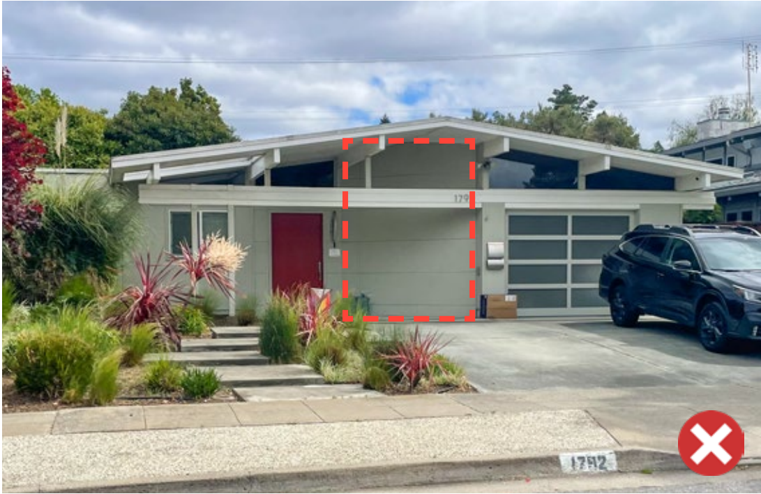
Figure 20: Enclosing carports and openings above carport walls (outlined in dotted red line) is prohibited.
