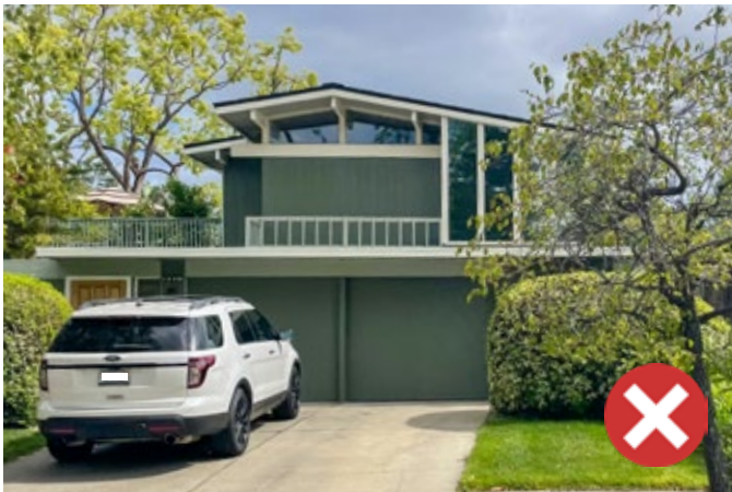
Figure 46: This addition not set back from the front facade and has a floor height that is taller than the original house.
