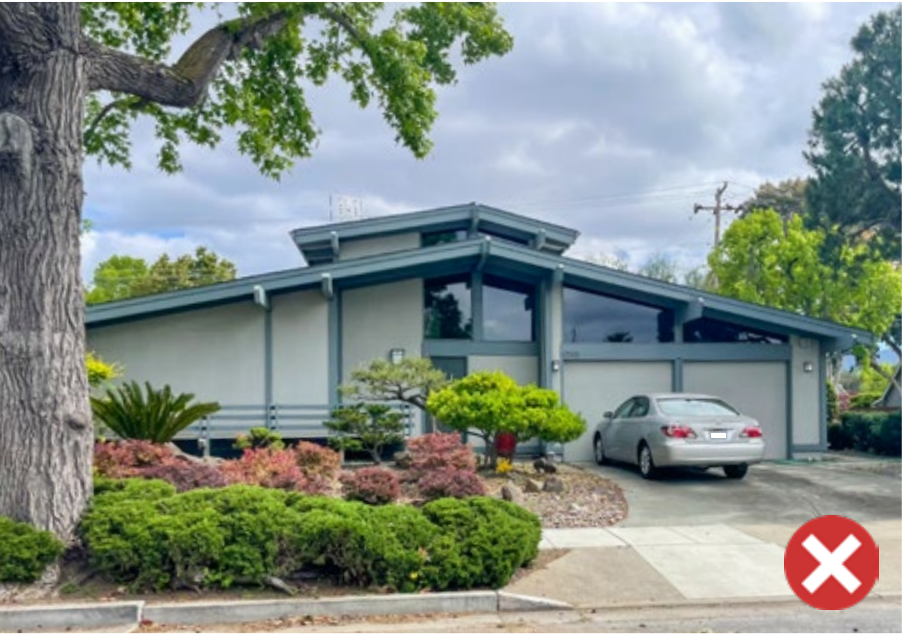
Figure 49: This atrium cover is too tall.
