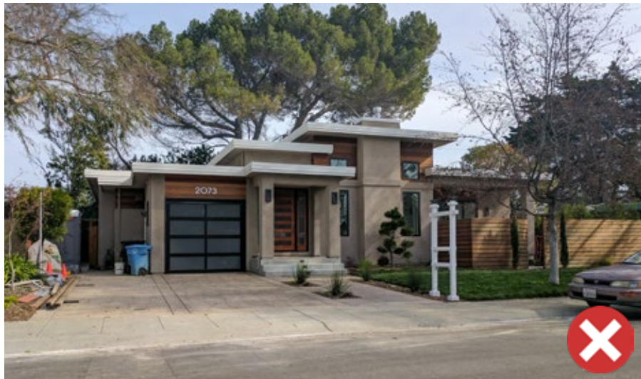
Figure 53: An example of a new house with compatible massing, contemporary style and flat roof, but too many diverse volumes. The portico at the front entry and modulated front facade are also not appropriate for an Eichler neighborhood.
