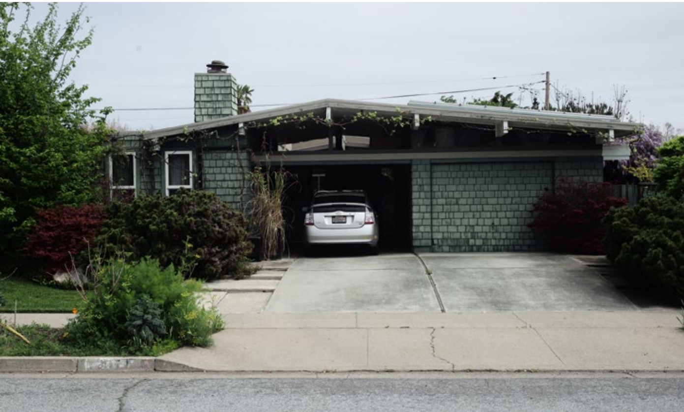
Figure 51: This altered Eichler residence has non-original painted shingle cladding. While some Eichler houses have wood shingles in select locations, painted shingle cladding across all facades is not original.
