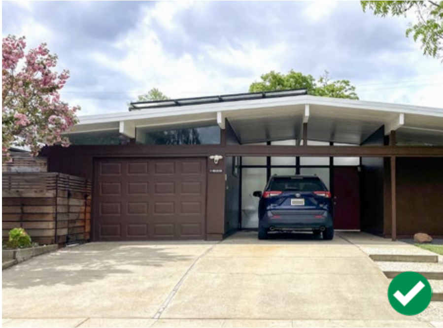
Figure 61: These rooftop solar panels do not rise substantially above the roofline, are parallel to the roof plane, and are minimally visible from the street.
