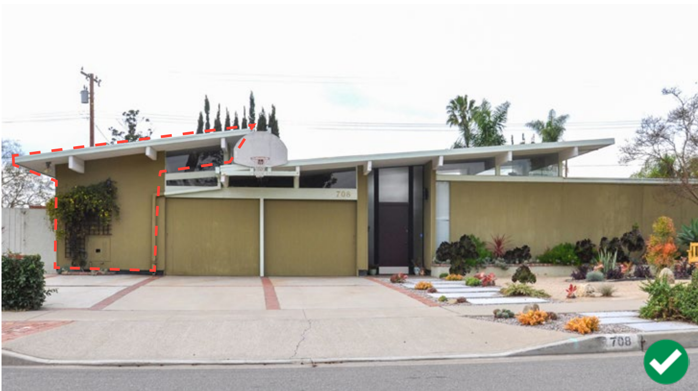
Figure 43: Side addition (outlined with dotted line) using the same roof form and slope as the original building. Setting this addition back from the main house’s front facade would have further increased its compatibility.
