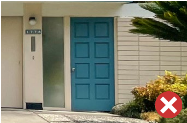
Figure 32: Replacement front entry doors with raised panels are prohibited when visible from the street.
