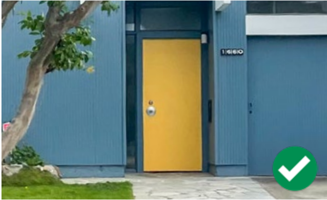
Figure 28: Maintain and repair original front entry doors that are visible from the street.
