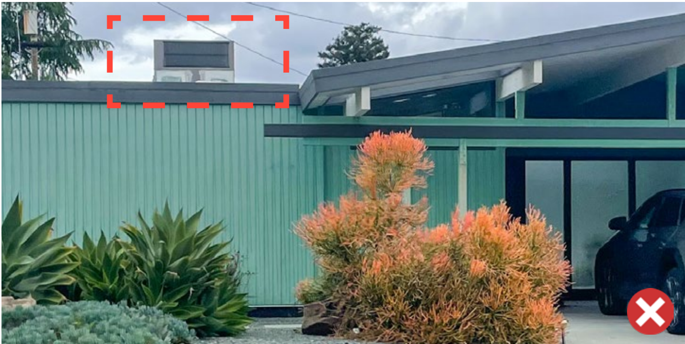
Figure 42: Roof-mounted mechanical equipment must be installed on the rear half of the roof to minimize visibility.
