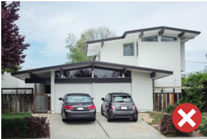
Figure 47: While this addition is set back and has a low-pitch roof form and appropriate cladding and windows, the floor heights are too tall.
