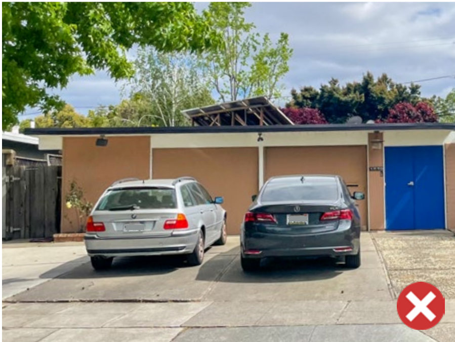
Figure 62: These rooftop solar panels rise noticeably above the roofline and are highly visible from the street.
