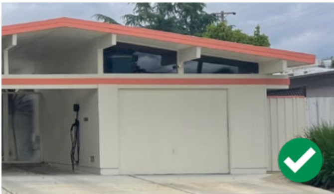
Figure 22: Preserve and maintain original garage doors.
