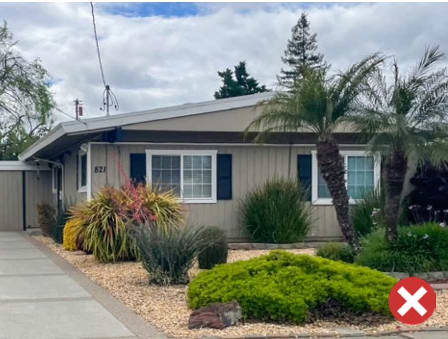
Figure 39: Vinyl windows, windows with divided glazing, and shutters are prohibited.
