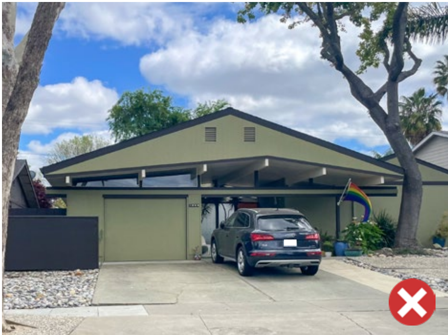
Figure 9: Raising a roof above its original height is prohibited.
