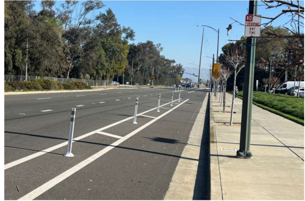
Right: New protected bikeway on Matrix Boulevard, upgraded with one-time grant funds.
