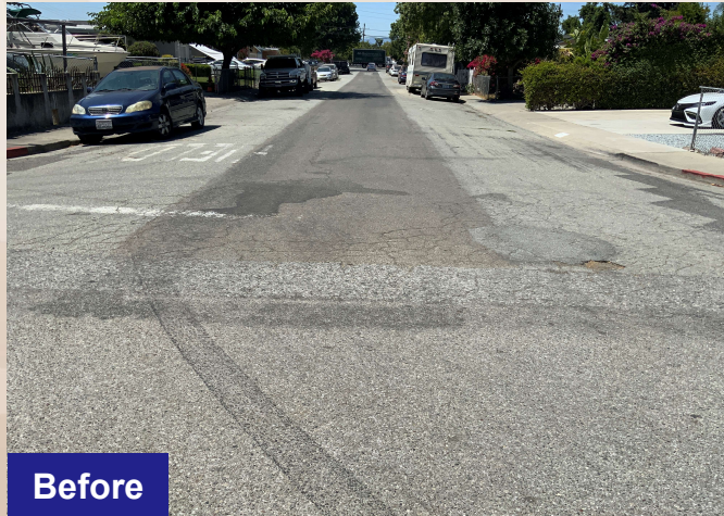
Berrywood Dr 2025 Resurfacing
