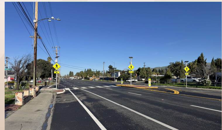
White Rd, Post-Resurfacing 2025
