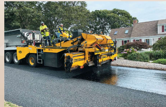
Application of Cape Seal Treatment
