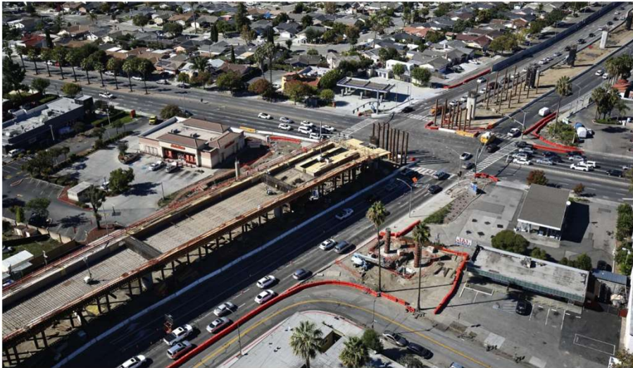
Bridge falsework south of Story Road
