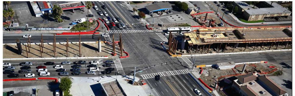
Bridge falsework supports in ground north of Story Road
