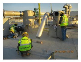
Contractors completing digester pipe installation.
