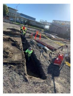
Contractor hand digging to expose utilities for the Facility Wide Water System Improvements Project
