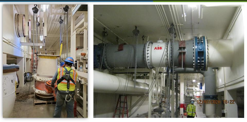
Contractor replacing flow meters in the Return Activated Sludge (RAS) pipe gallery.
