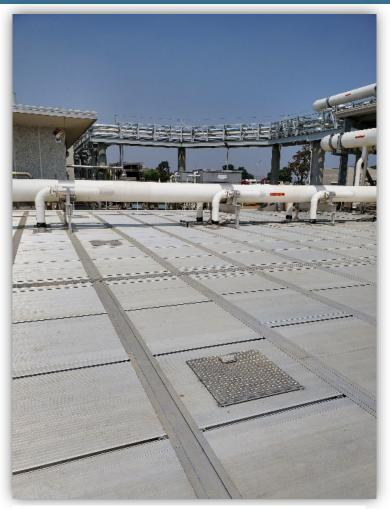
Dissolved air flotation thickener (DAFT) covers and odor control piping.
