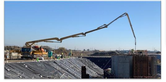
Concrete placement for influent structure walls.
