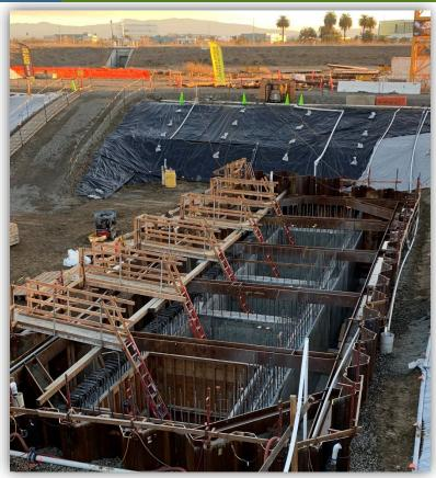
Construction of raw sewage pump station wet wells.
