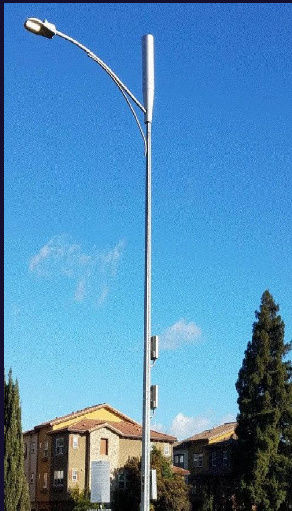
Small Cell installed on a streetlight
