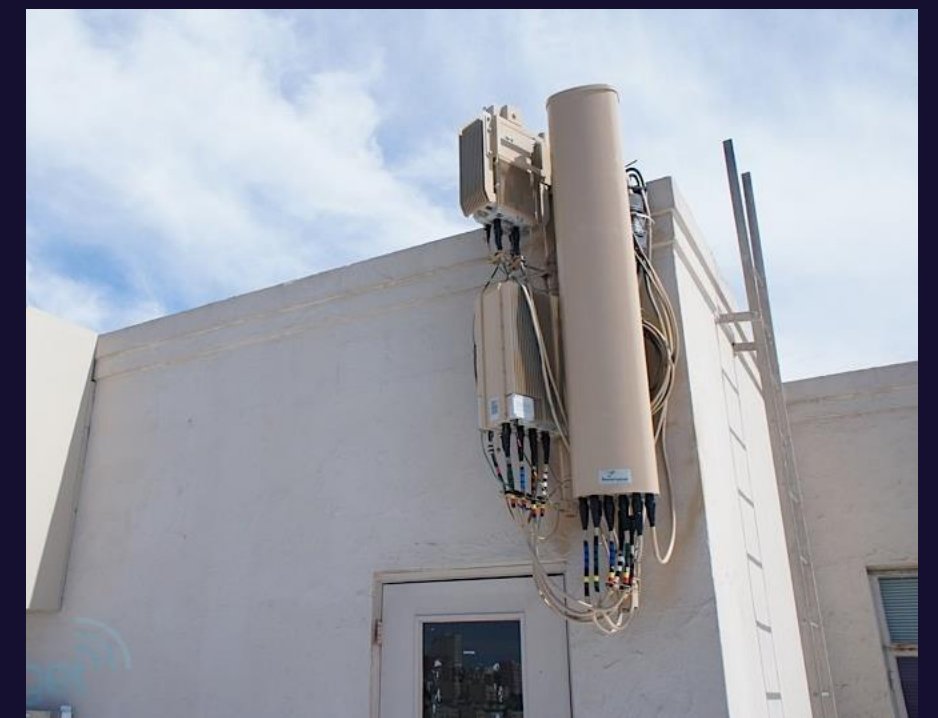
Macro Cell installed on a rooftop
