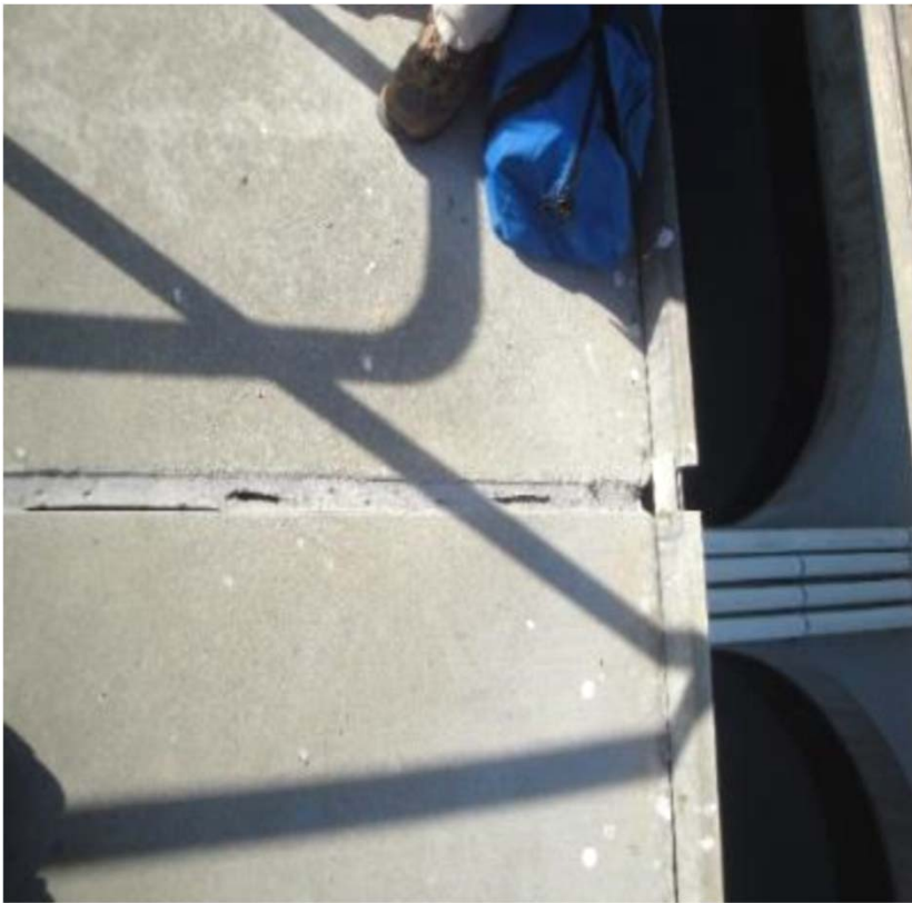
Existing Expansion Joint with Cracks
