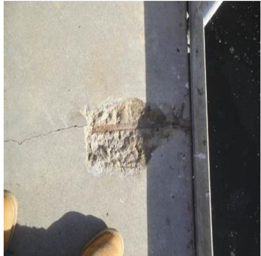
Concrete Spalls
