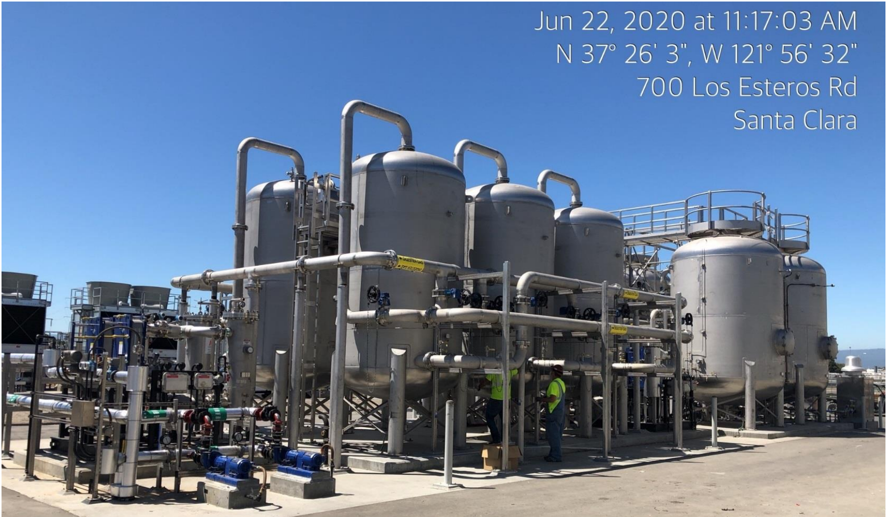
Contractor Starting Up Gas Treatment Skid
