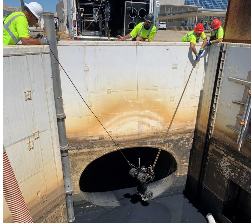
Contractor Clearing Sludge from the 87-inch X 136-inch Pipe, and Conducting Pipe Inspection Using a Remotely Operated Vehicle (ROV)
