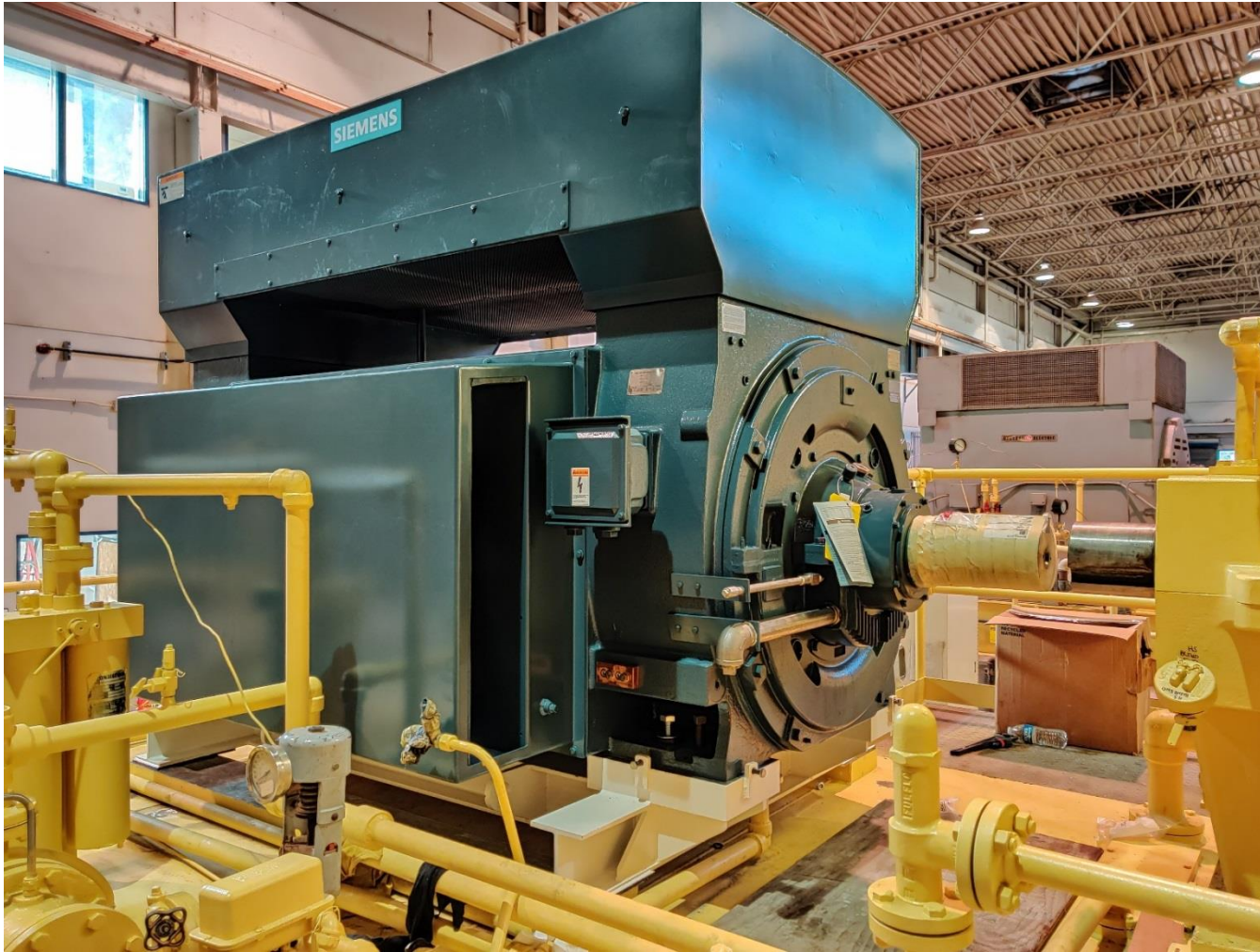
New Electric Motor Installed for Blower (PAB 2)
