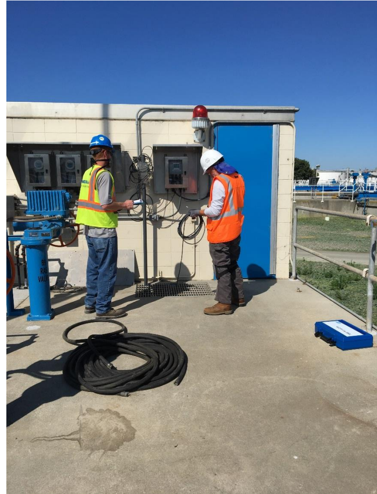
Contractor Conducting Functional Testing on Various Instruments
