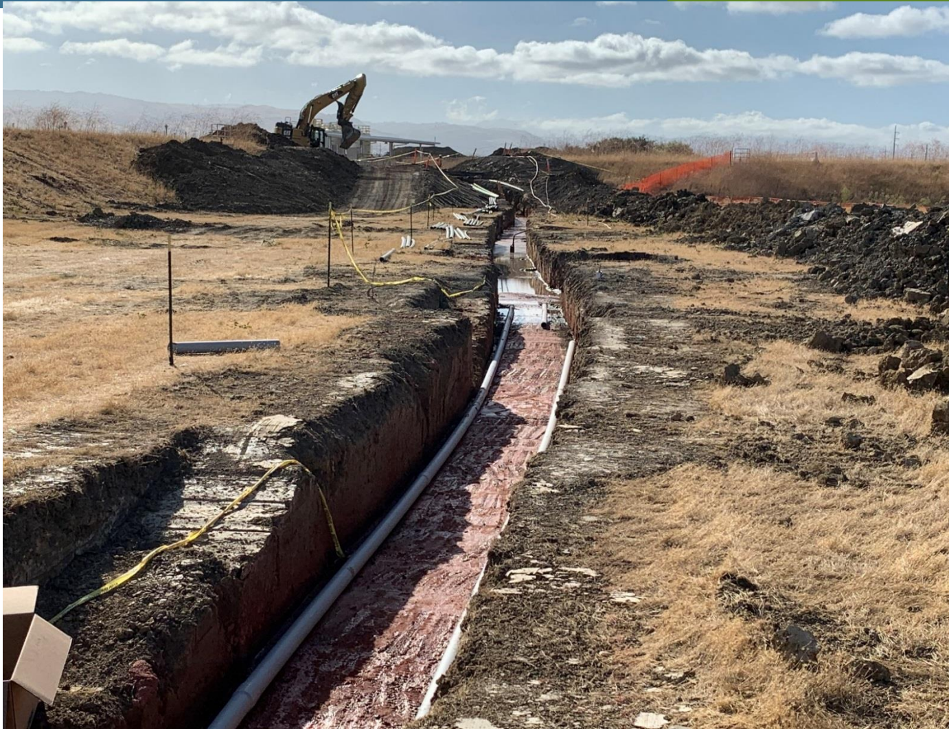
Temporary Electrical Duct Bank Reroute
