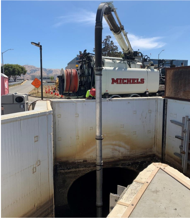
Contractor Clearing Sludge from the 87-inch X 136-inch Pipe, and Conducting Pipe Inspection Using a Remotely Operated Vehicle (ROV)
