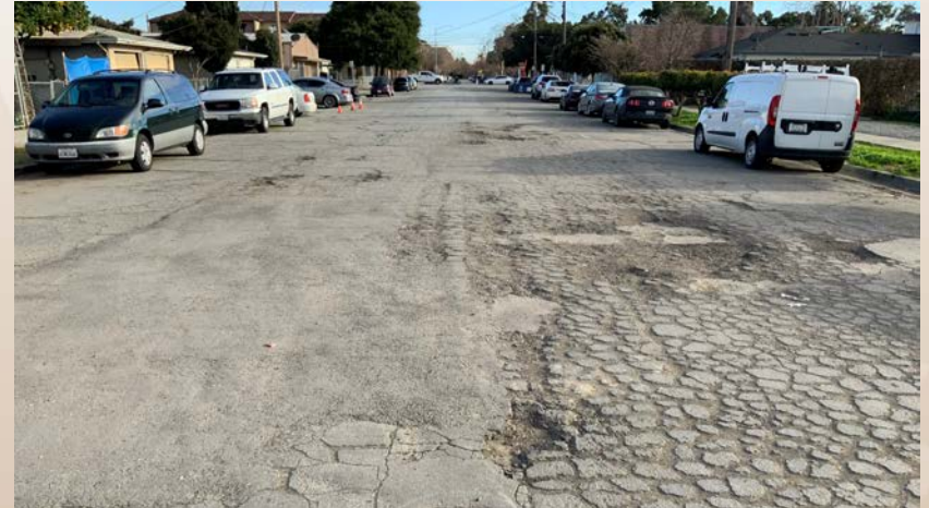
Eighth St: PCI 23, 1990 Chip Seal
