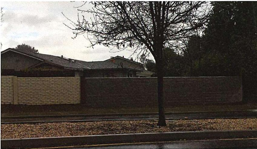
And this photo shows a section of wall where the homeowner didn't need a permit, and was allowed to simply replace the damaged panel with cinderblocks, reinforced with steel rods. Replacement time was about three weeks.
