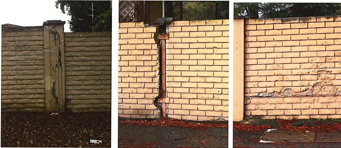
In the center photo, above, you can see the concrete panel on the left has fully separated from the steel connecting post. This is not uncommon and it is becoming more and more common to see entire panels missing. In some cases, residents have replaced the damaged panels with plywood. There are several examples of this around the City, but here is one example:
