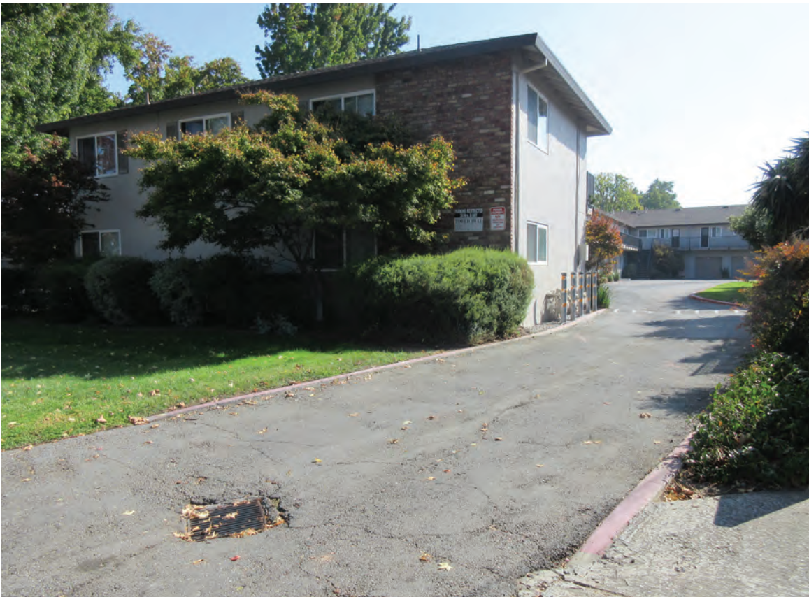
2 - View of the adjacent multi-family building to the east.
