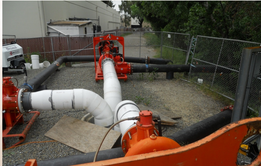
Temporary Pumping at Charcot near Coyote Creek
