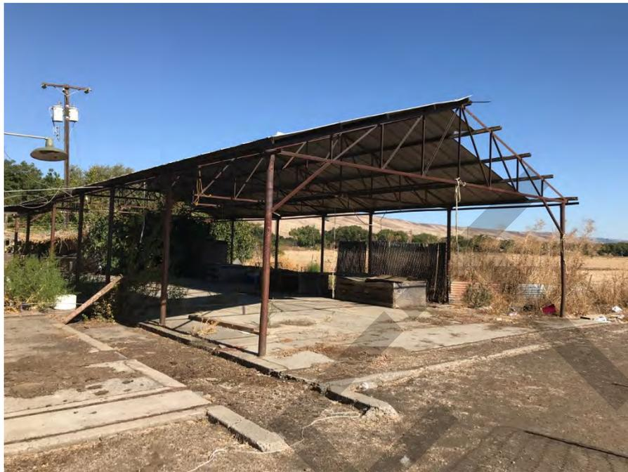
Southern portion of the Emado Compound. Second tin roofed pole barn south of eastern cinder block building with concrete pad with missing portions of the roof.
