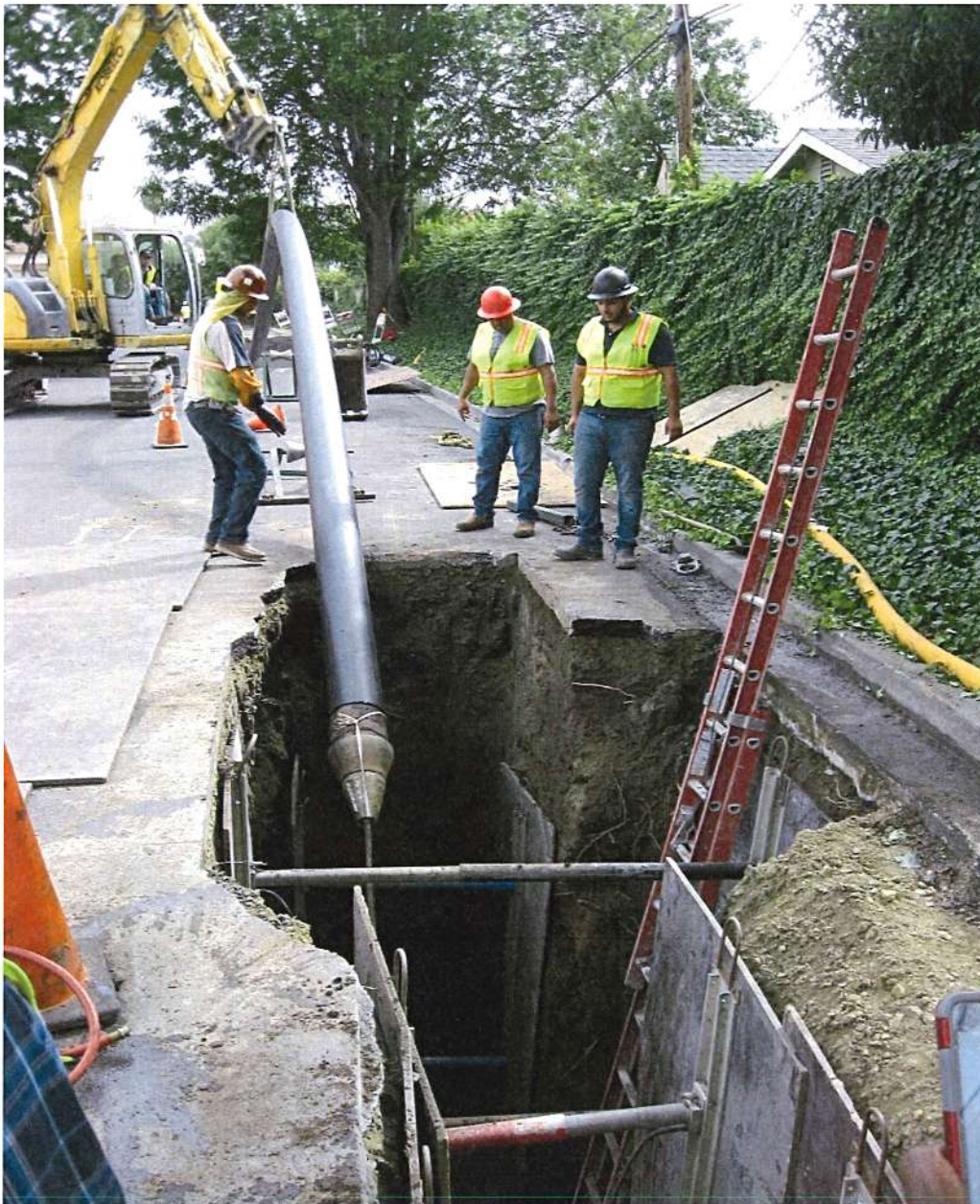
Trimble and Amberwood Sanitary Sewer Improvement Project - Pipebursting
