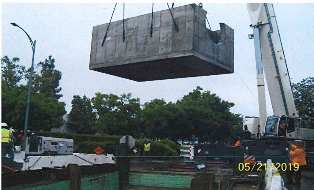
Large Trash Capture Device Installation
