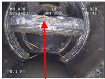
Replace Corroded Butterfly valves
