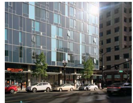
DO and DO NOT - Operable windows enhance livability and sustainability. Shading devices would have reduced the potential for glare.
