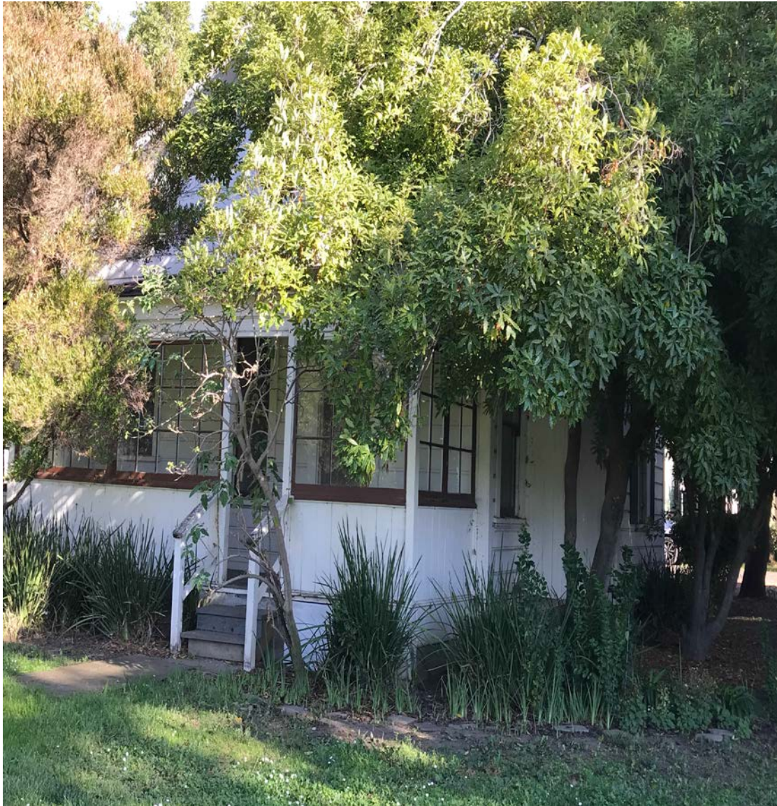
Photograph 5 Chiechi House, History Park San Jose View: Rear façade, added porch that has been enclosed. Vertical board siding on the half wall of the porch Camera facing: SE Date of Image: September 2018
