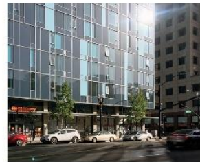
DO / DO NOT - Operable windows enhance livability and sustainability. Shading devices would have reduced the potential for glare.
