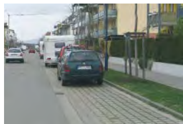
Permeable paving for street parking strips reduces rain water run-off.
