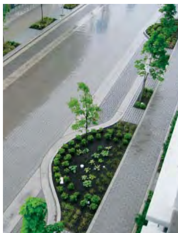
Provide generous bulb-outs for street trees and pay attention to detailing for curbs, drainage, and pavement.
