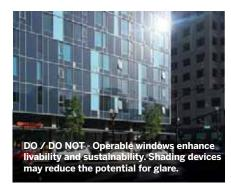
c. Respond to the building's orientation by varying the fenestration on different facades. Use architectural elements such as shading devices or balconies to regulate solar gain on southern and western facades with passive solar design. Technological solutions such as windows with variable opacity may be used as an alternative.
