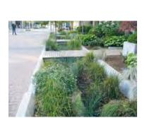
Bioswales retain rain water and reduce the impact on the storm water system. If designed well, they can improve and green the streetscape.
