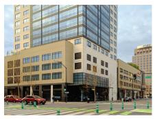
**D0** - Treat the *facade* of an exposed parking garage with materials and design similar to the rest of the building and extend the tower facade to ground level (see Section 4.3.1).
