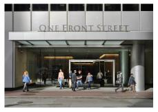
**DO** - Create visibility into the lobby to welcome pedestrians. A recessed entry and canopy provide protection from the elements when necessary.
