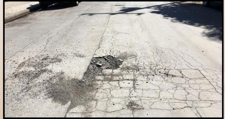
Failed (Below PCI 25) – Pacific Ave PCI 23
