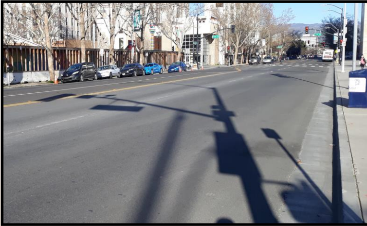
Good (PCI 100 to 70) – Santa Clara St. PCI 91
