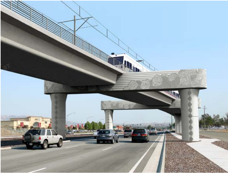
Median to side running transition near Tully Road
