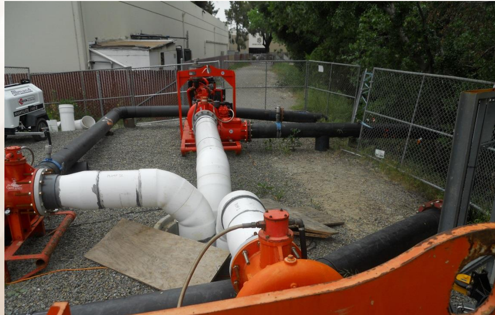
Temporary Pumping at Charcot near Coyote Creek
