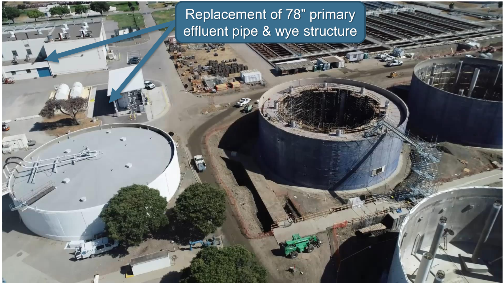
Digester Upgrades: Rehabilitation of Digesters 5-8 and replacement of 78" primary effluent pipe and wye structure
