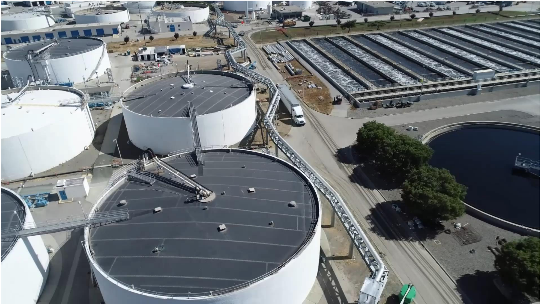
Digester Upgrades: New elevated pipe rack and gas piping.
