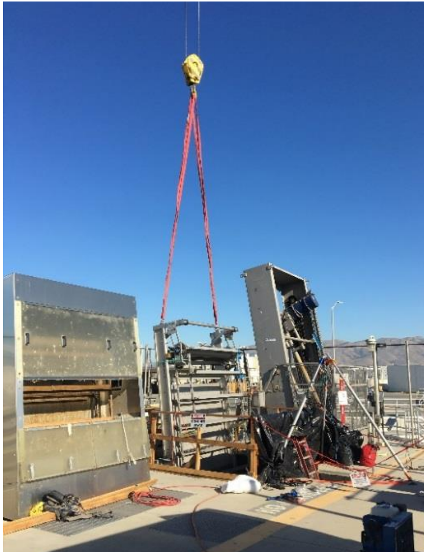
Headworks Critical Improvements: Newly installed bar screens for Headworks #2
