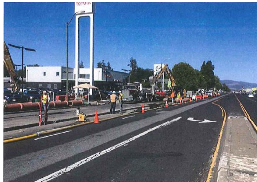
Stevens Creek Blvd Pipe Installation
