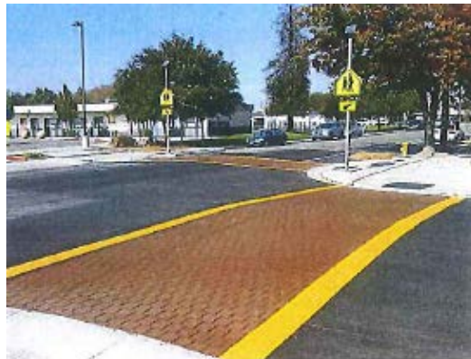
Five Wounds Brookwood Terrace Pedestrian Improvements: After Photo
