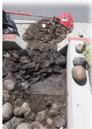
Remove Sediment Build-Up and Debris from Inlet and Forebay
