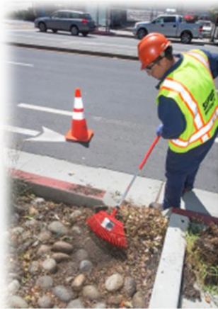
Remove Sediment Build-Up and Debris from Inlet and Forebay
