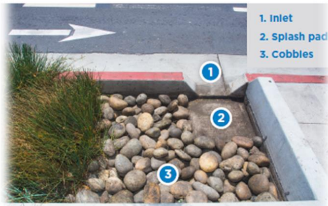
Remove Sediment Build-Up and Debris from Inlet and Forebay
