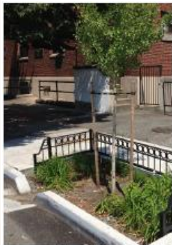
Stormwater Tree Wells
