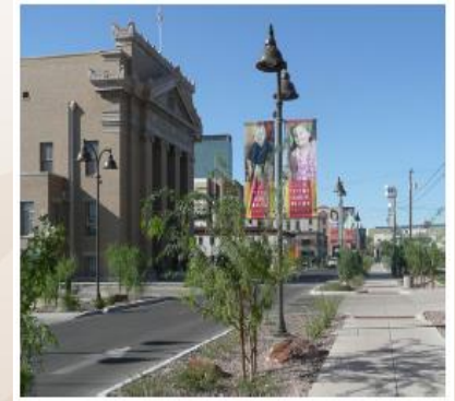
Infiltration & Flow Through Planters
