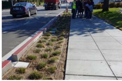
Bioretention in Sidewalk
