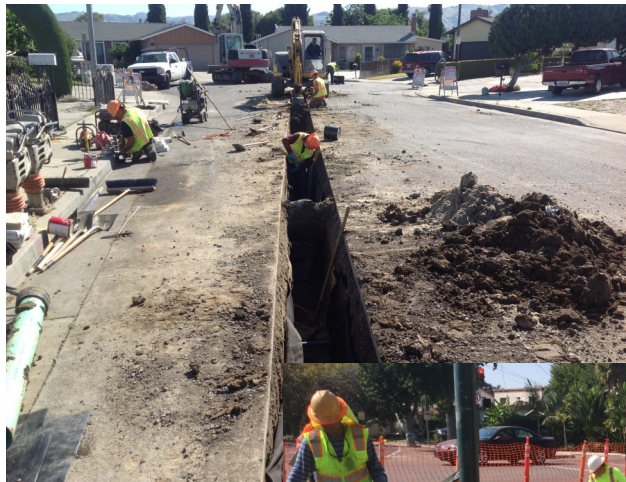
Tolbert Ct. Sanitary Sewer Cast Iron Replacement
