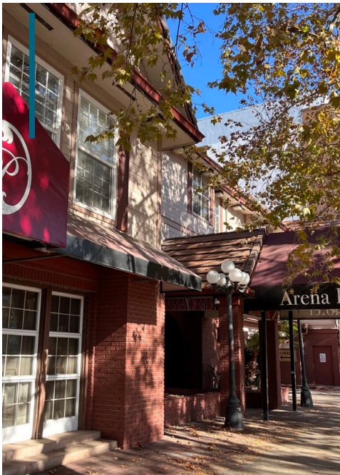
Hotel/ Motel Sheltering
