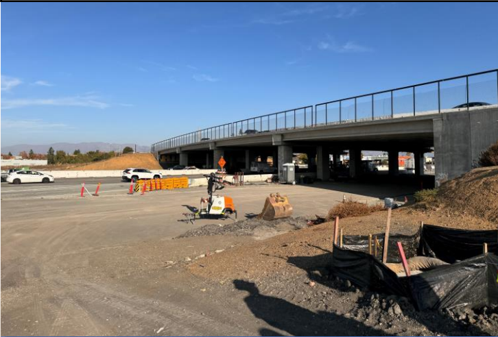
Vehicular Overcrossing Bridge over US 101
