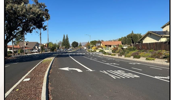
Ruby Av, post-resurfacing 2024
