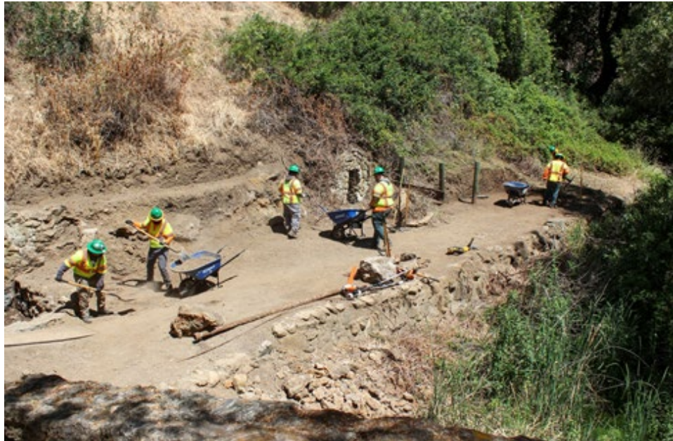
Figure 2 Resilience Corps Members Working at Alum Rock Park
