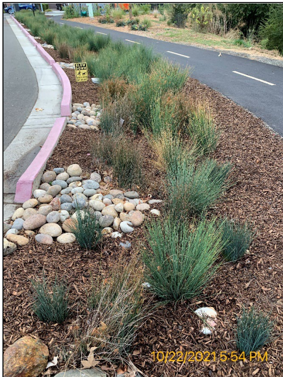
Bioretention Area along the Guadalupe Mines Trail.
