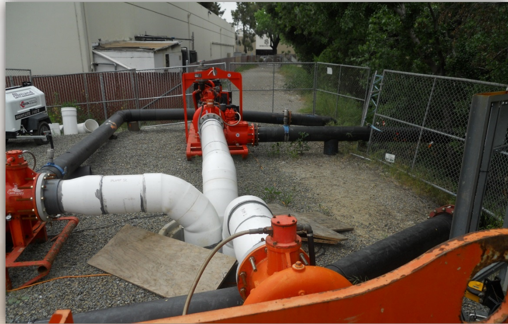
Temporary Pumping at Charcot near Coyote Creek
