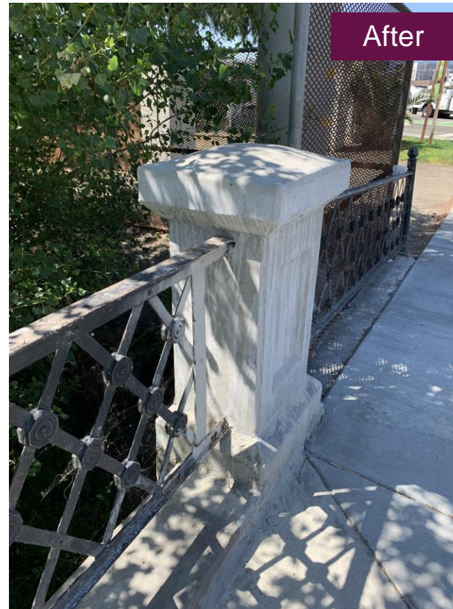
San Fernando St Bridge
