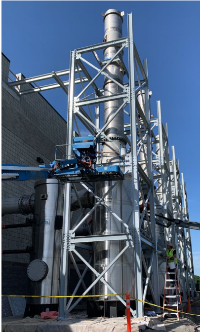
Figure 1: Cogeneration Facility Heat Exhaust Stacks Structural Steel
