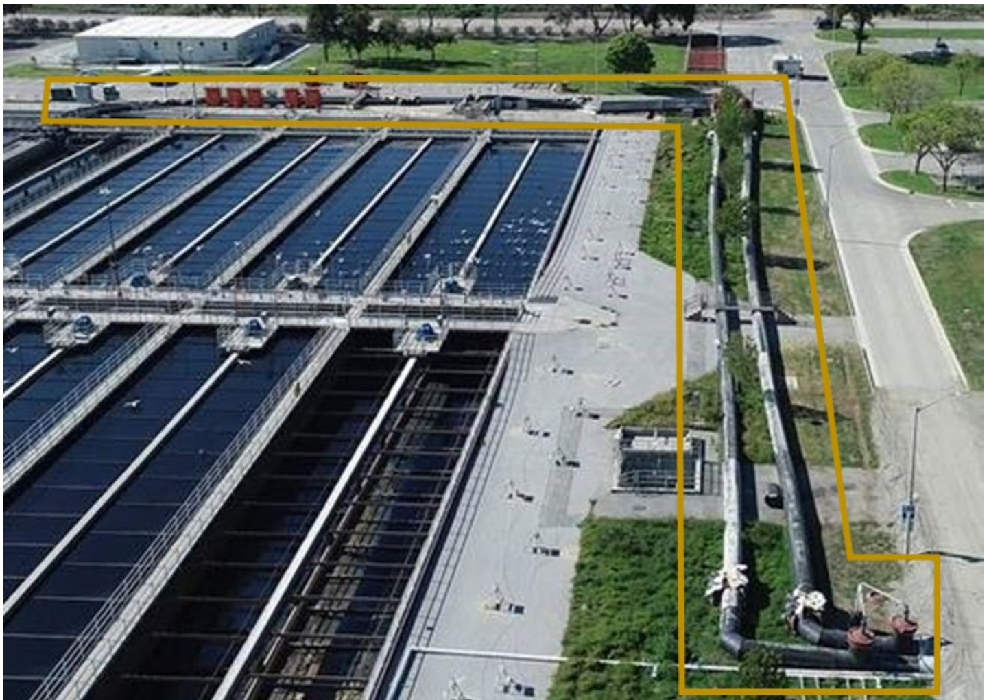
Figure 5: 78-Inch SES Reroute System Outlined in Orange
