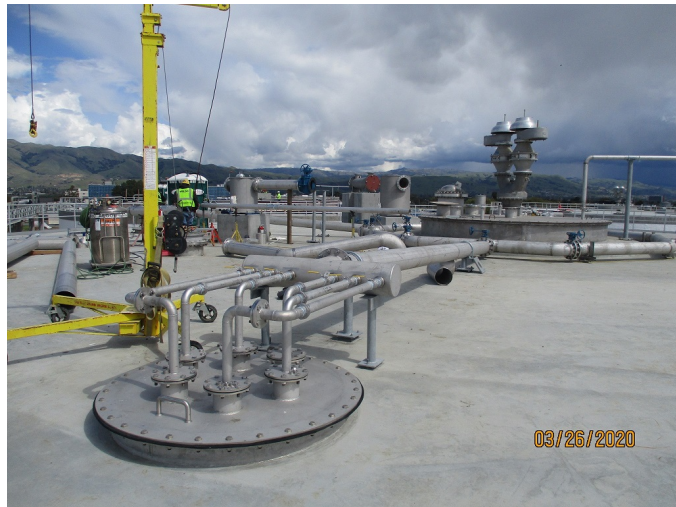
Figure 11: The Digester 5 gas withdrawal system is comprised of injection piping shown nearest, and pressure relief valves and digester gas separators in the distance. The digester gas will be used by the new Cogeneration Facility engines to generate electricity and heat for the RWF.
