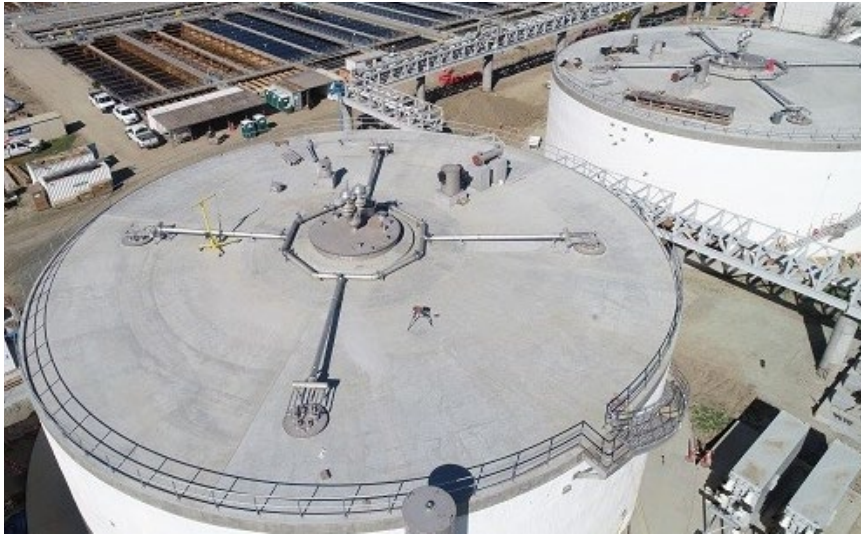
Figure 1: Aerial view of the Digester 5 (left) and Digester 6 (right) gas withdrawal system
