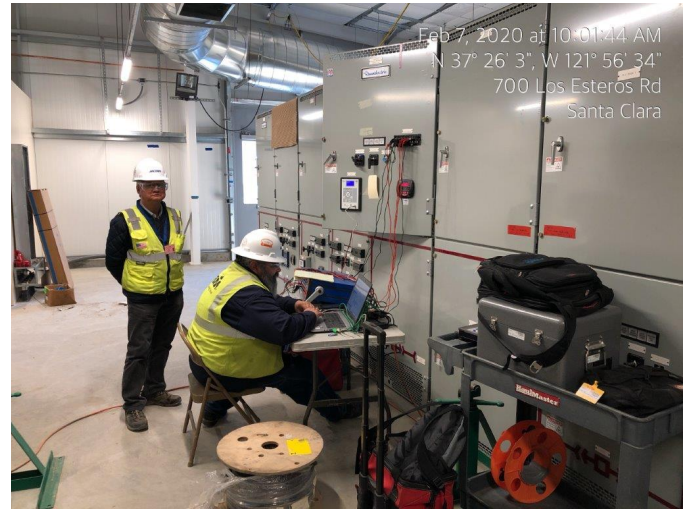
Figure 7: The electricity generated by the new engines will use this medium voltage (4160 Volt) switchgear to distribute power to equipment throughout the RWF. The workers shown are testing the wiring and protective relay settings prior to putting the switchgear into service.
