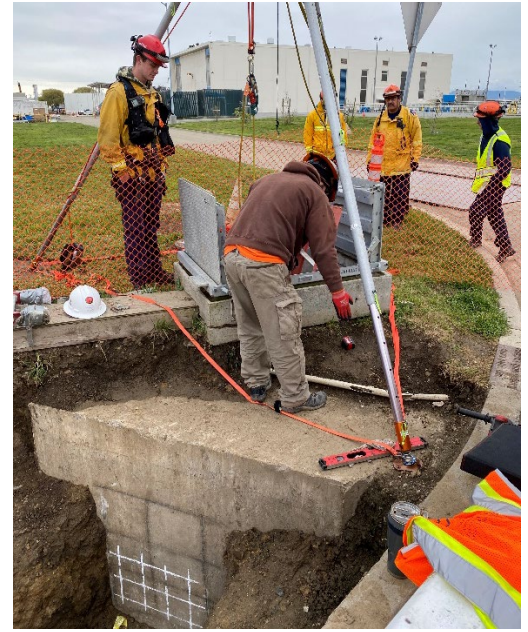
Figure 3: The contractor prepares the existing electrical conduit system maintenance access point for additional conduit connections. The existing rebar locations are marked on the outside of the concrete junction structure to guide new conduit positioning.
