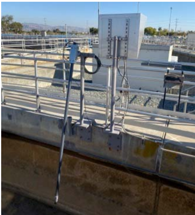
Figure 7: New Total Suspended Solids Sensor and Transmitter at the Secondary Mix Liquor Channel
