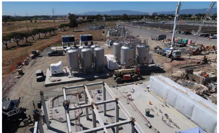
Figure 3: Bottom left: Pipe support structure under construction. Middle: Hydrogen sulfide and siloxane removal equipment. Middle right: Electrical ductbank concrete pour.
