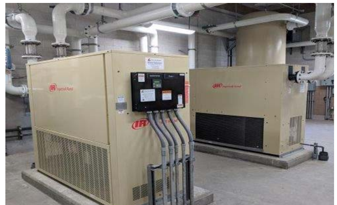
Figure 9: Refrigerated Air Driers
