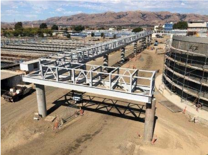
Figure 2: Pipe rack system and Digester 6
