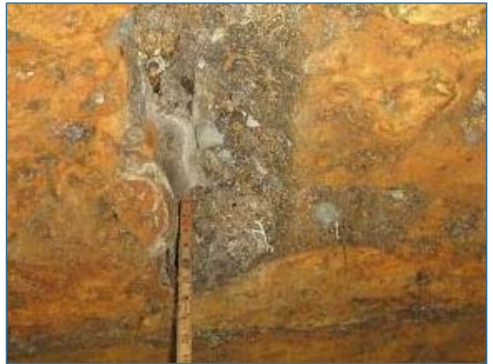
Figure 6: Crown corrosion pocket of 87-inch SES Pipeline
