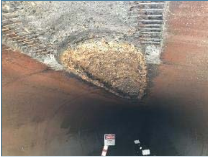
Figure 5: Crown corrosion of 87-inch SES Pipeline
