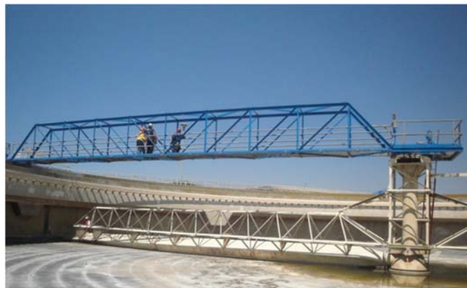
Figure 4: Clarifier Interior and Mechanism
